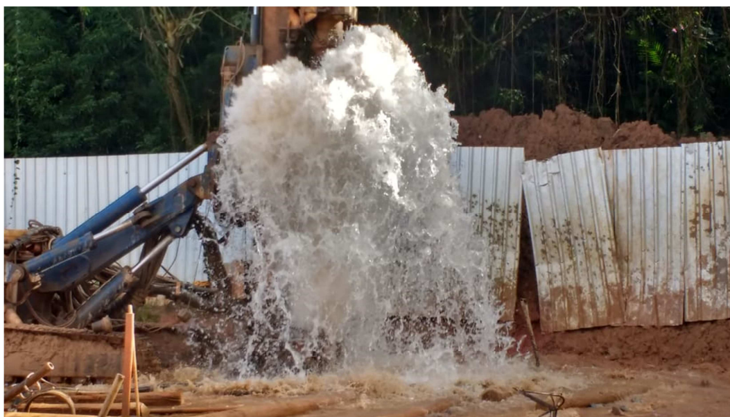
Figure 3. Artesian well during the drilling phase
