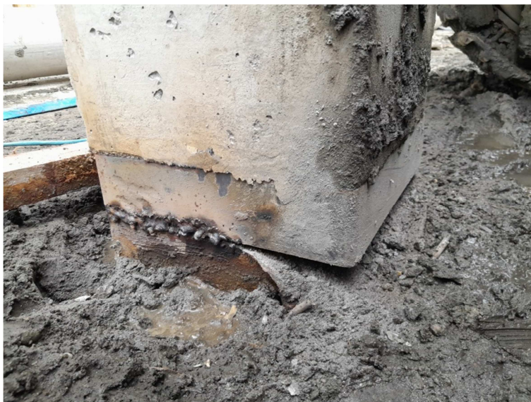
Figure 2. The welding area of the 29.5cm-square pile
