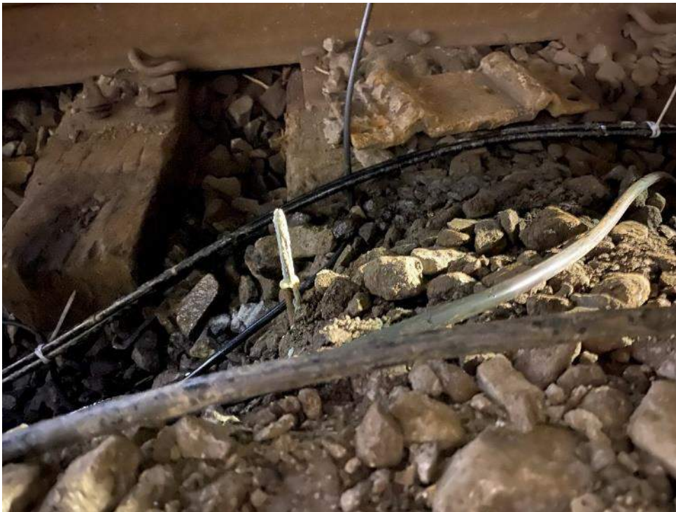
Figure 16 - Packer injected with structural silicate resin
