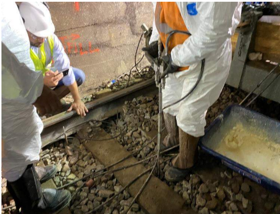
Figure 14 - Injection of material with two-component injection equipment
