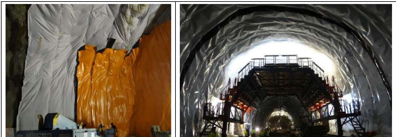
Figure 13 - Examples of drainage fleece and membrane in a metro cavern and in a rail tunnel. In the latter with a curved perimeter of about 30 m there will be the need for 12 to 15 km of membrane welds per running kilometer of tunnel. If membrane leakage should occur and enter the tunnel via a shrinkage crack in the concrete, the actual leakage location will not be detectable, so post injection will likely fail
