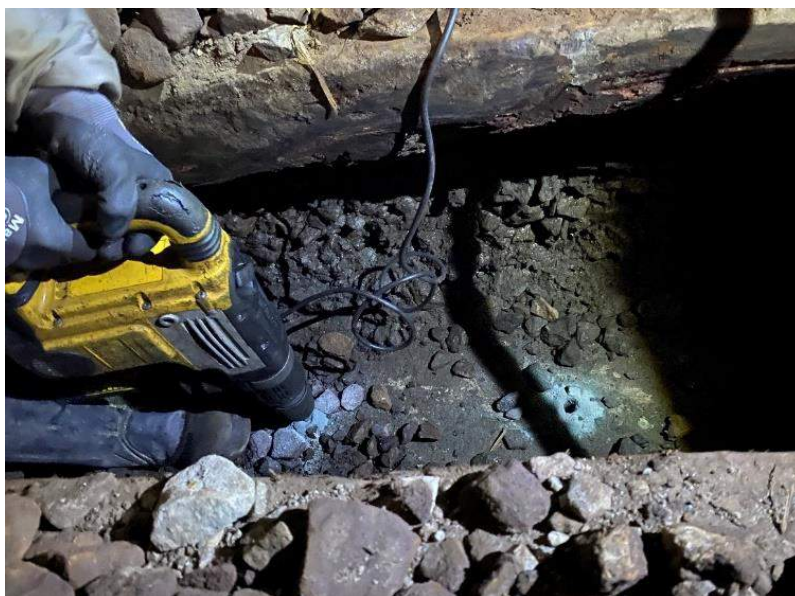
Figure 10 - Drilling the slab below the ballast
