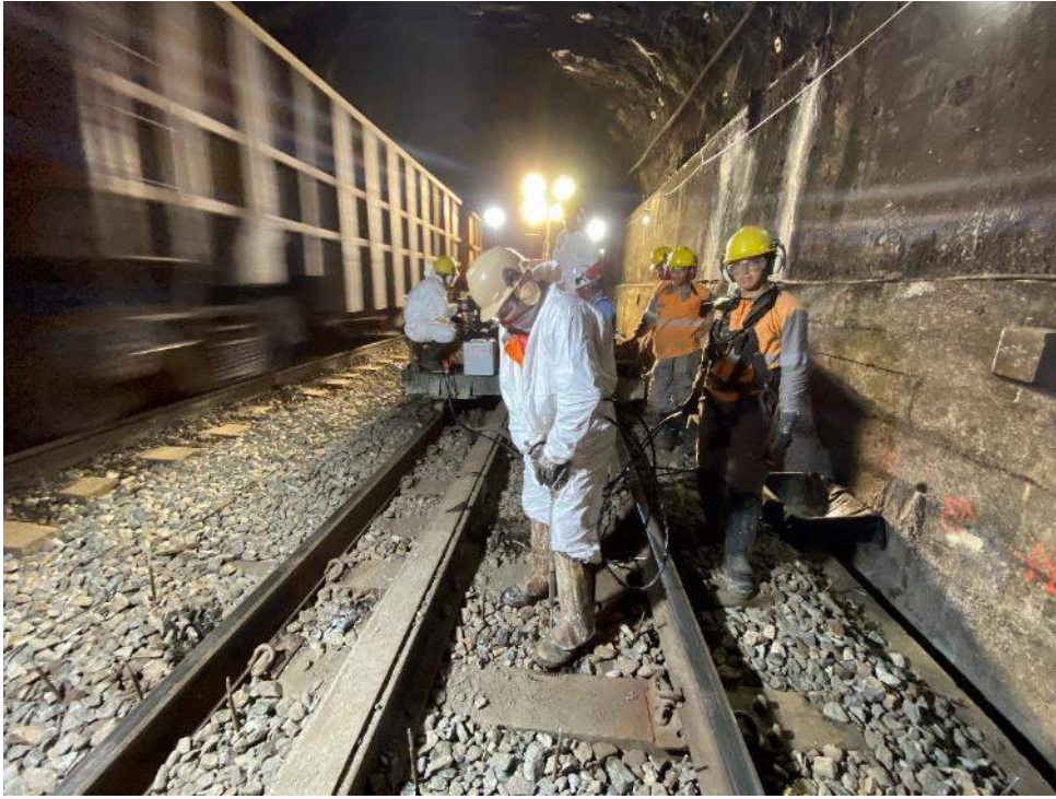
Figure 15 - Injection of the structural silicate
