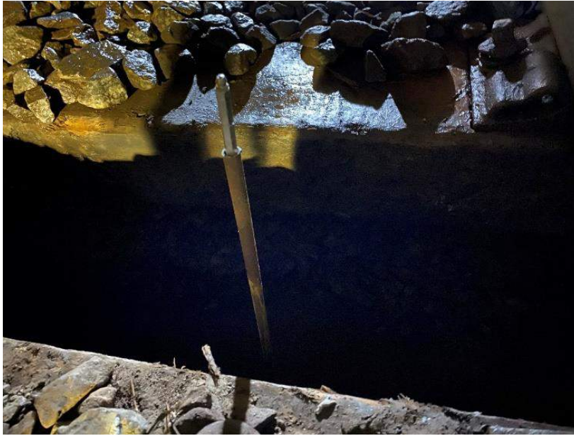
Figure 11 - Injection packer and tube installed
